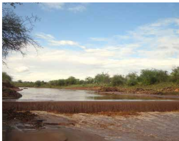
Above: A sand dam is under construction in Kajiado County, Kenya. Below: A completed sand dam in Kajiado County, Kenya.
